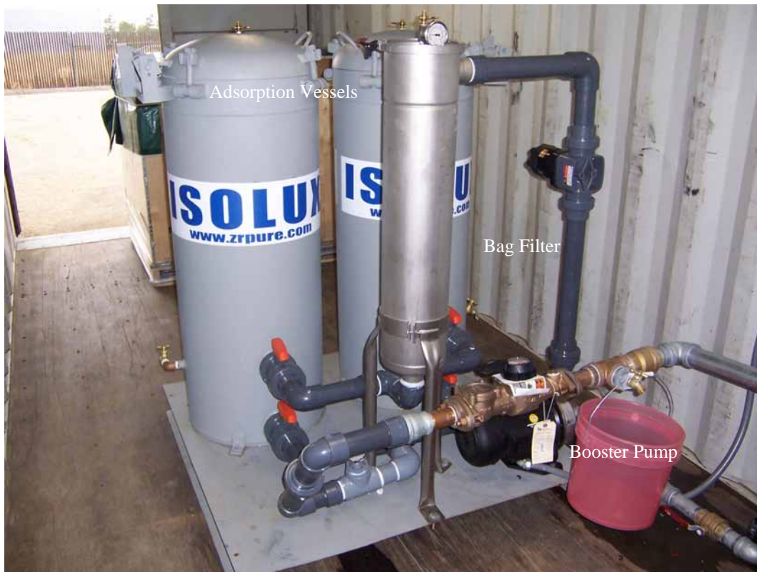
Figure 4-7. Isolux™ Adsorption Module at GHCS D
