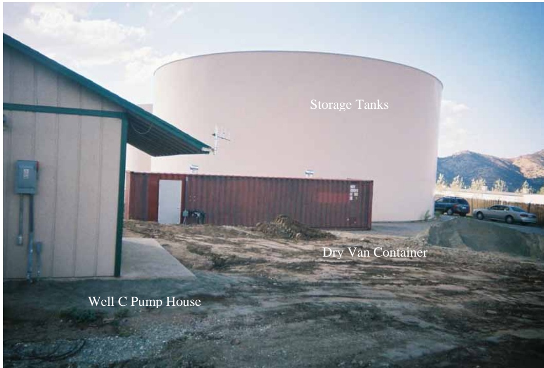
Figure 4-2. Storage Tanks, Well C Pump House, and Dry Van Container
