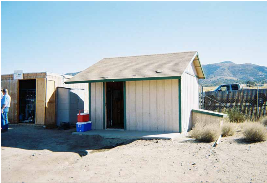
Figure 4-1. Well C Pump House
